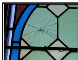
Pressure Cracks
